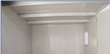
Building reinforced with metal columns and beams
